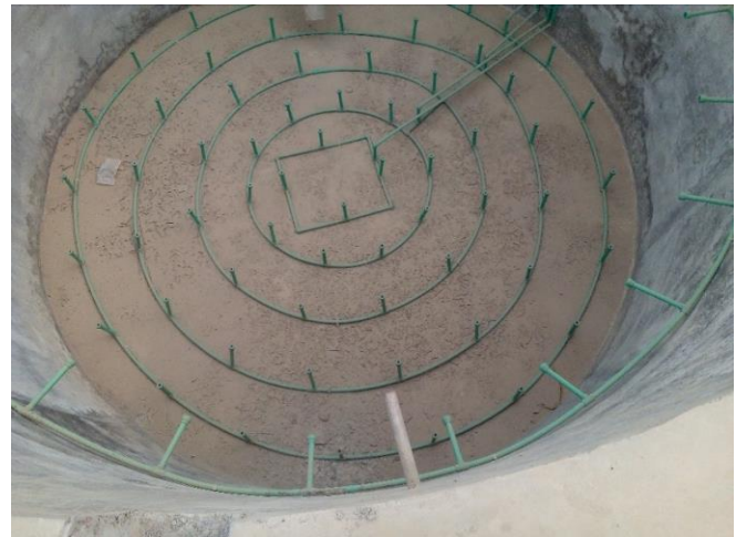
Figure 4. Installation of reverse blasting technique inside the digester.
