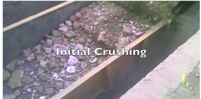
Fig. 6: Initial Crushing, of Rubble Waste
