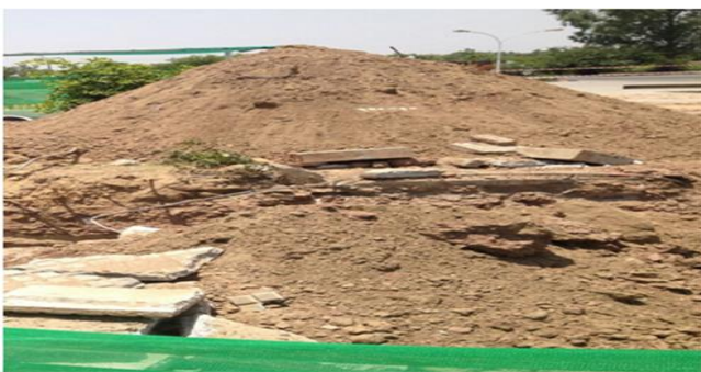
Fig. 4: The Demolition Waste that was Produced after the Demolition
