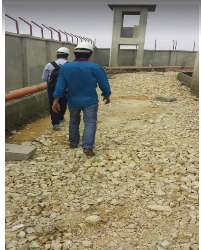
Fig. 1: Site Survey prior to Demolition
