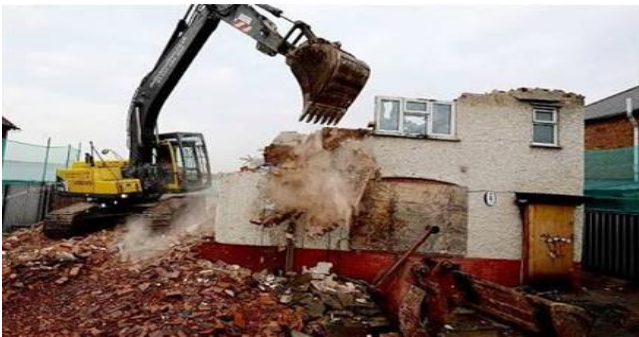
Fig. 3: A View of Barracks being Demolished
