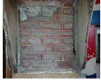
Fig 27: Damaged Plaster
