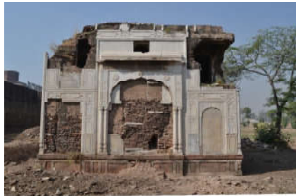
Fig 12: Design of niches exposed brick on the north side Source: Author
