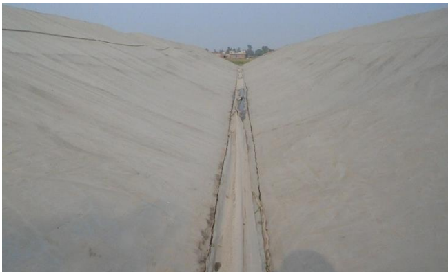
Figure 10. Rainwater harvesting drainage channel/gutter
