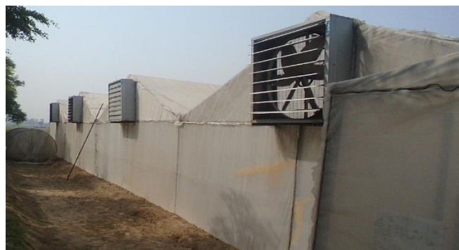
Figure 8. Co-axial exhaust fans installed in each bay of greenhouse
