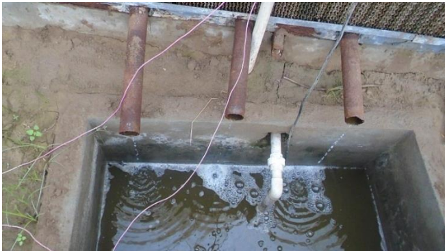
Figure 9. Drainage sump (Reservoir)
