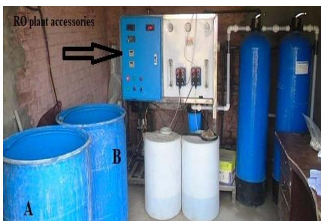
Figure 12. RO plant accessories, A: micro-nutrient tank, B: macro-nutrient tank
