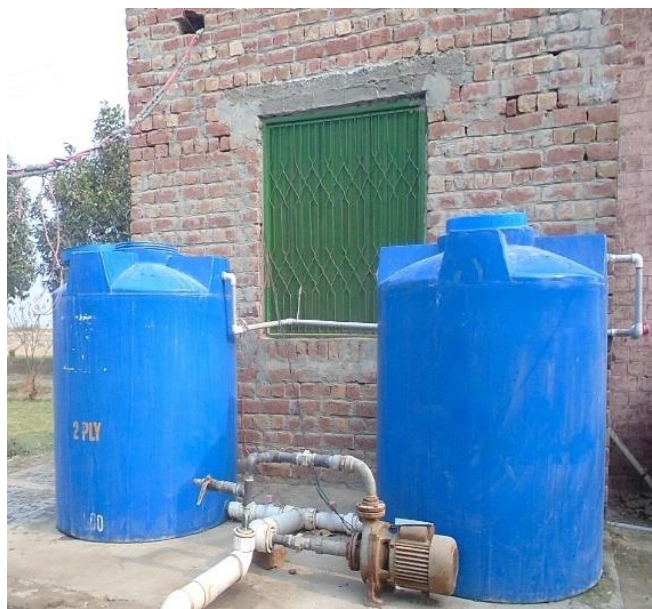
Figure 14. RO water storage tanks for recipe preparation
