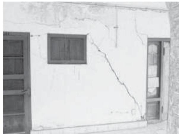
**Fig. 2.** View of Exterior cracks
