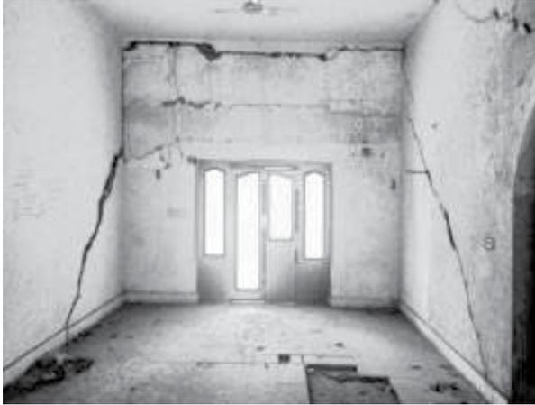
**Fig. 3.** View of Interior cracks
