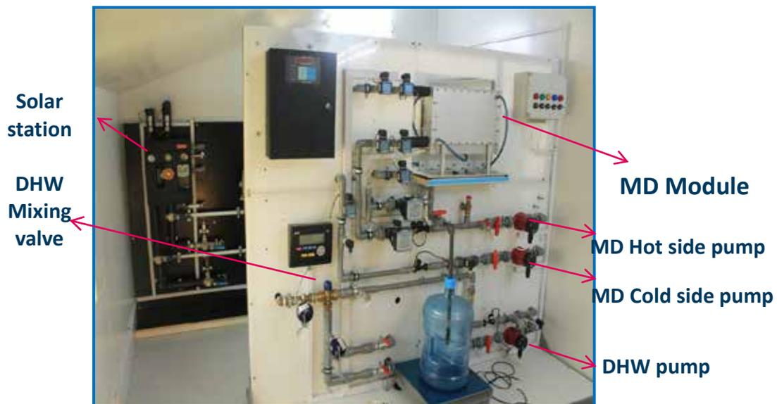
**Fig. 5.** MD system with solar station.
