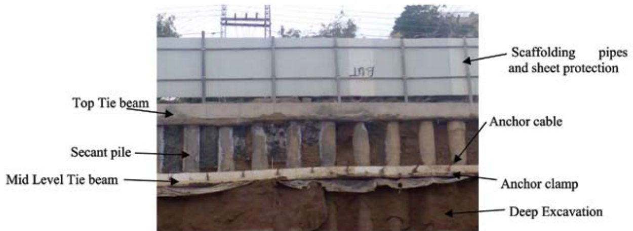
Fig. 3. Components of secant pile earth retention system.
