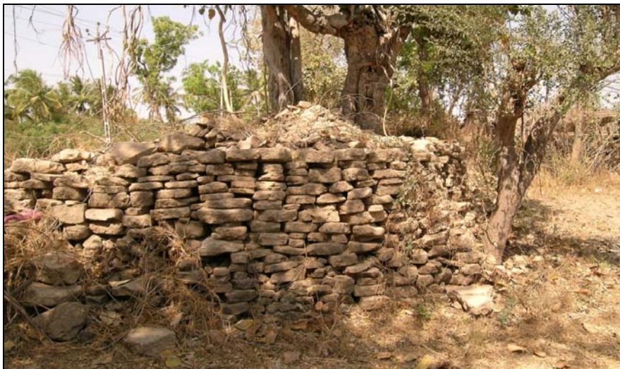
Figure 5: The Pile of Remains of Disturbed Structures, Talli
