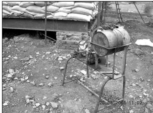
**Plate 3:** Oil reservoir pump and pressure gauge
